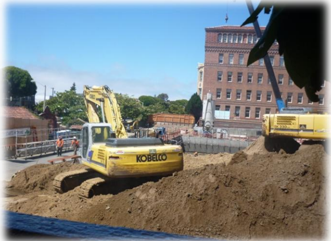
Hospital Development Site
