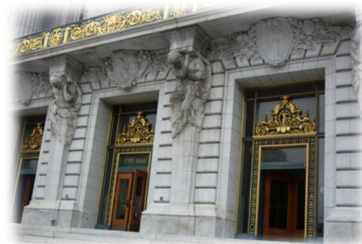
San Francisco City Hall (entrance)
