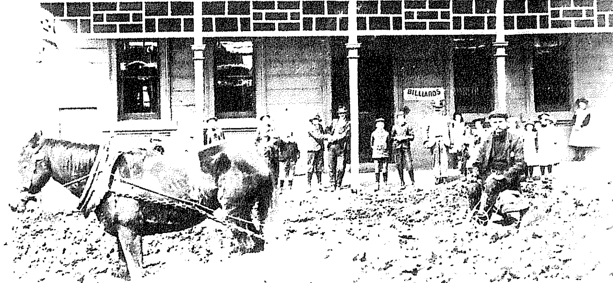
A SAMPLE of Korumburra mud, into which this horse sank a foot outside the old Austral Hotel. Challenges like this were commonplace to road-making surveyors and engineers.
